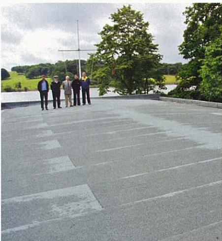
The completed roof at TS Derby Sea Cadet Unit
