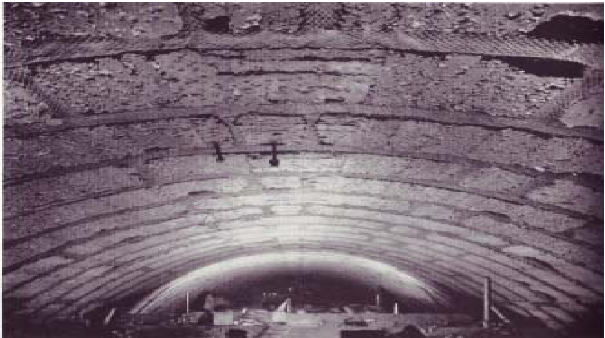
Waterproof sheeting on London Underground tunnels
