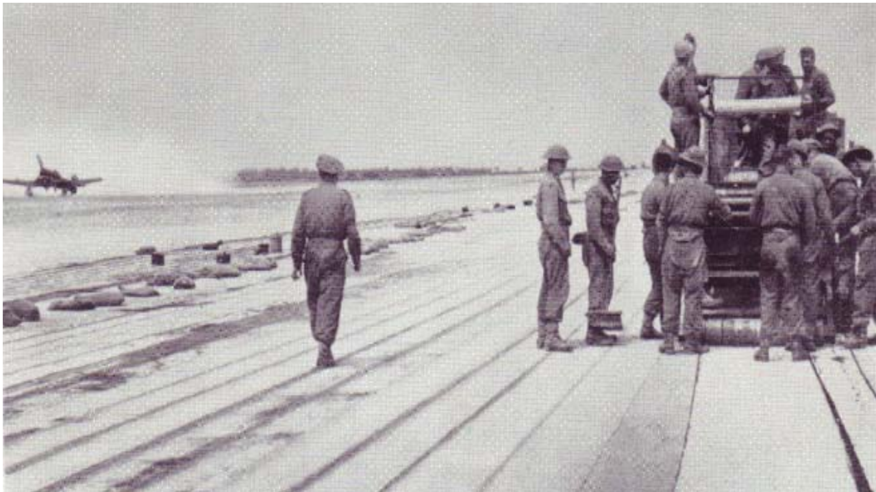
Royal Engineers laying Briggs' sheeting on a temporary runway in France
