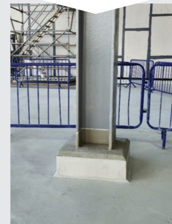
Each of the numerous rooftop column and plinth details are being finished with liquid waterproofing by BriggsAmasco to ensure a watertight finish.
