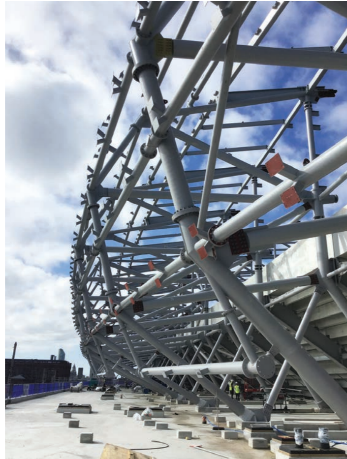
BriggsAmasco is laying around a 1,000 tonnes of mastic asphalt on the first level perimeter roof of the new Bramley-Moore Dock Everton stadium. Once the company is finished in October 2023, the huge steelwork structure will be clad covering most of the roof area and the huge quantities of plant it will house to provide services for the up to 62,000 fans the stadium is designed to seat.
