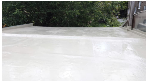
Image above shows the new leak free roof!
