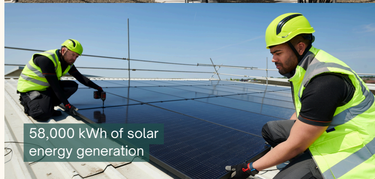
Over £1million of investment in electric transitioning
